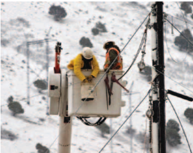
Limit the time workers are in dangerous situations. Hydro workers limit the time they work outdoors in cold weather.
