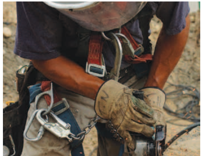
By wearing Personal Protective Equipment, workers can avoid many incidents. This worker is wearing a face shield to protect his face from sparks and flying dust. He is also wearing a fall prevention harness.
